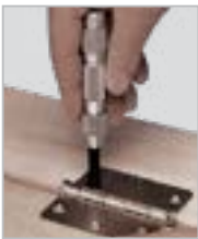
Punch being used to mark screw starting centres on a door frame
