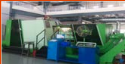
Multi-station Cold Forging Shop with equipment from NEDSCHROEF, Belgium, for manufacture of high volume automotive parts, sockets etc.
